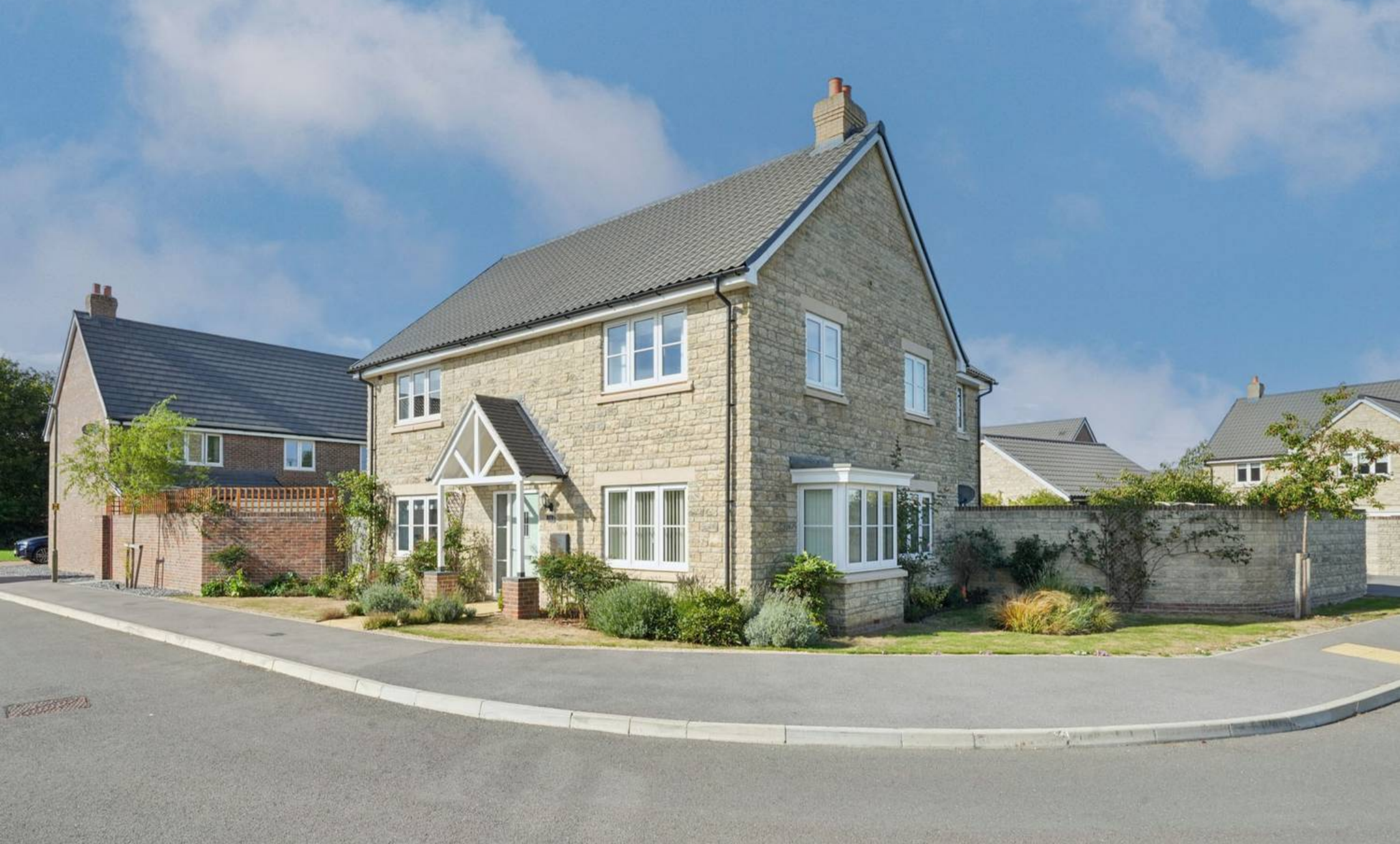
14 Pound Field Road, Aston
