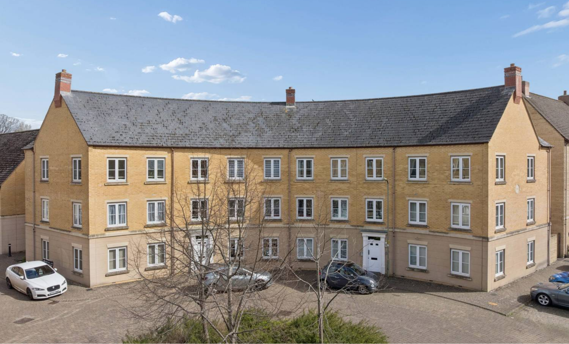
9 New Bridge Street, Witney
