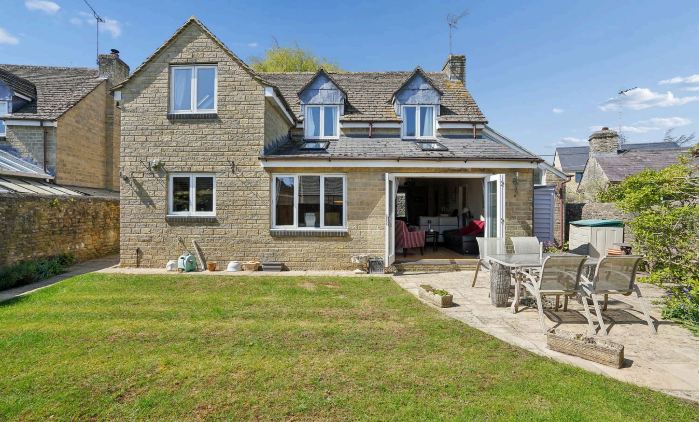
1a Well Lane, Curbridge
