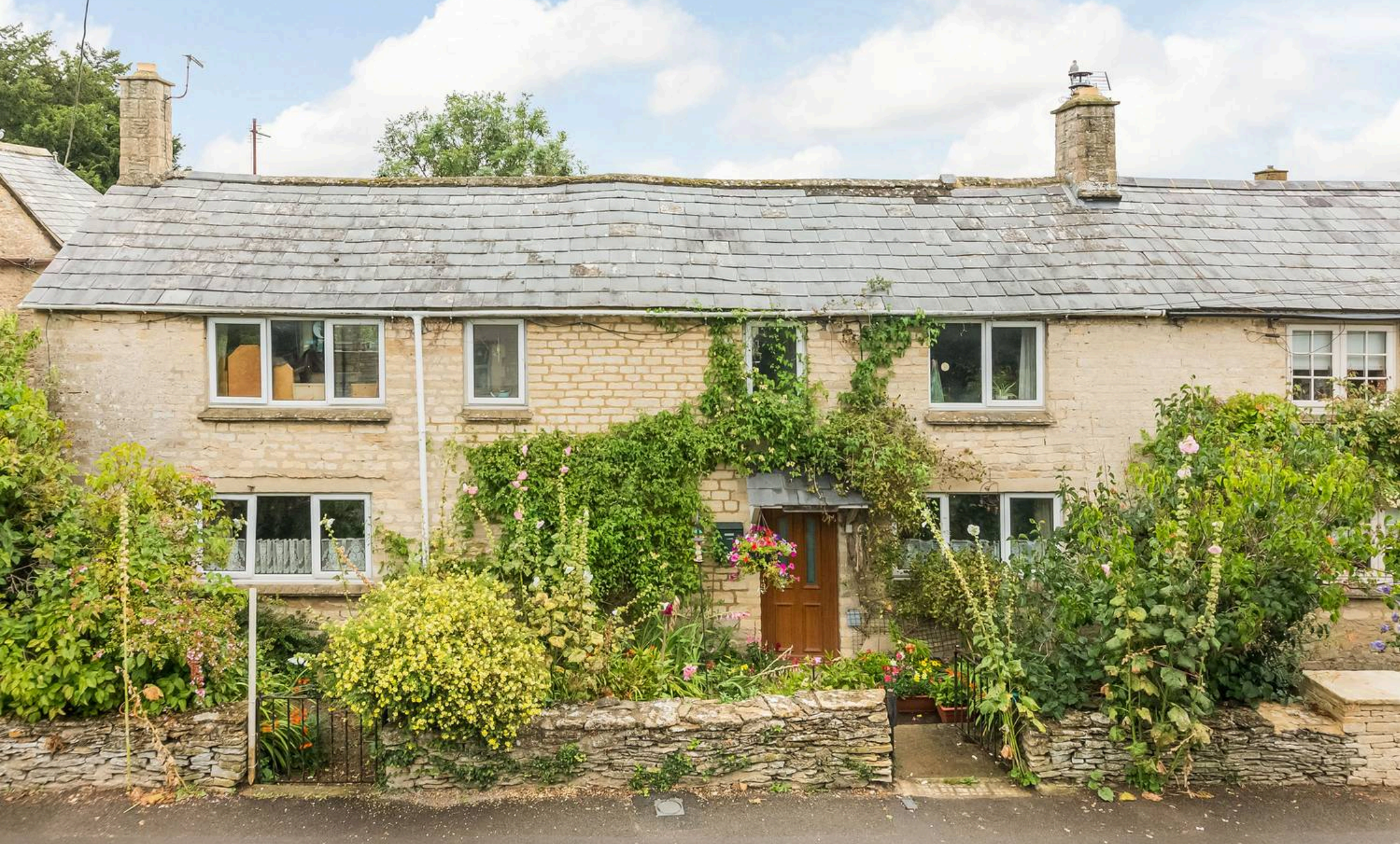
5 Station Road, Brize Norton
